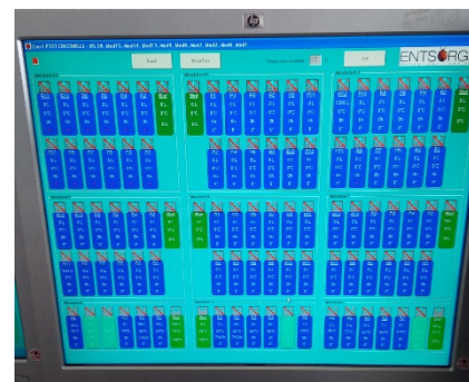
(3) H24/7 CONTROL SYSTEM
